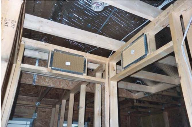
R.A.P. Transfer Grilles with baffles exposed
