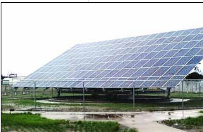
Nebraska Public Power District's photovoltaic solar energy system in Norfolk can generate up to 44 kilowatts of electricity an hour.
