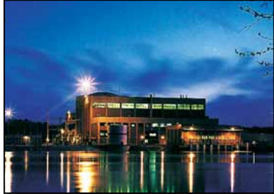
Fort Calhoun Station, 20 miles north of Omaha, has a generation capacity of 478 MW.
