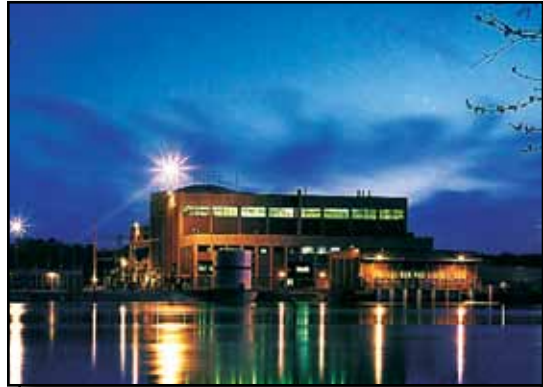
Fort Calhoun Station, 20 miles north of Omaha, has a generation capacity of 478 MW.
